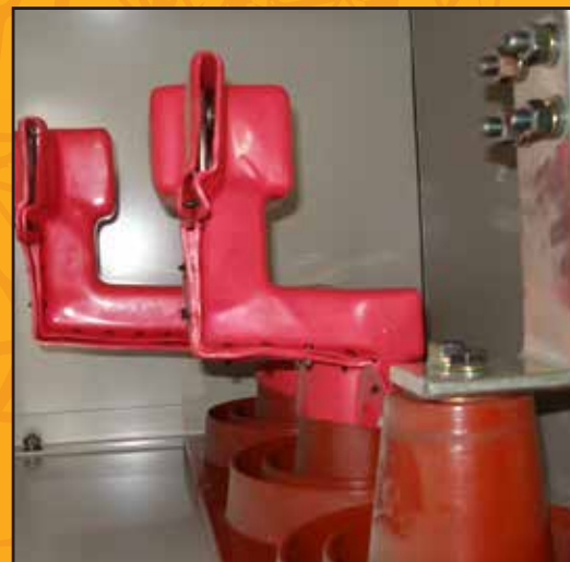
Control Panel with Shrouds
